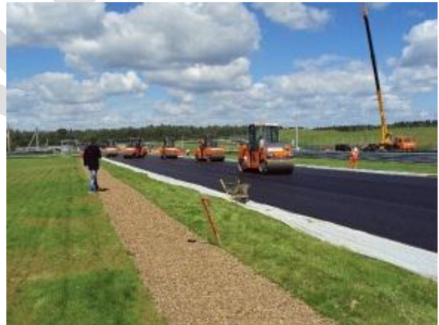
Rollers put final touches on pavement compaction at the Moscow Raceway
